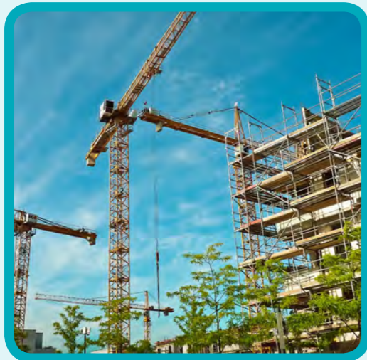
BUILDING UNDER- CONSTRUCTION
