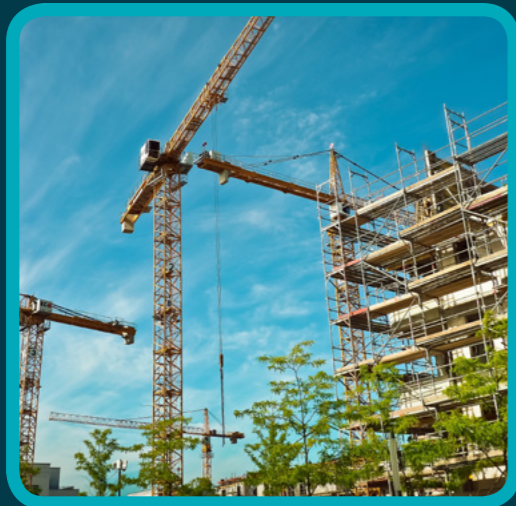
BUILDINGS UNDER CONSTRUCTION
